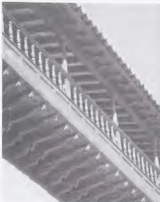
Buildings in the Canary Islands are known for their unique balconies, which are derived from North African and Spanish types; Tenerife, Canary Islands. Photographs by Graziano Gasparini. (From Armitano Arte 18.)
