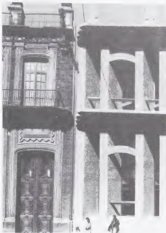
Remodel of the central office of the National Bank of Mexico (Banamex), Mexico City; Teodoro González de León, with Abraham Zabudovsky, 1986–88. (From México: Nueva arquitectura .)
